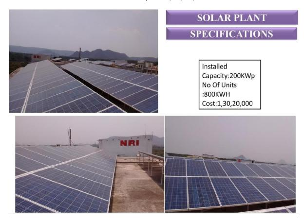
The solar roof tops/power system were installed on the two blocks of the institution named as MAIN BLOCK and EEE block .with installed capacity 105KWp and 95KWp Respectively The power generation by the solar roof tops connected to the grid tie inverters in each block for feeding power to the local APCPDCL ,Substation Grid system .
